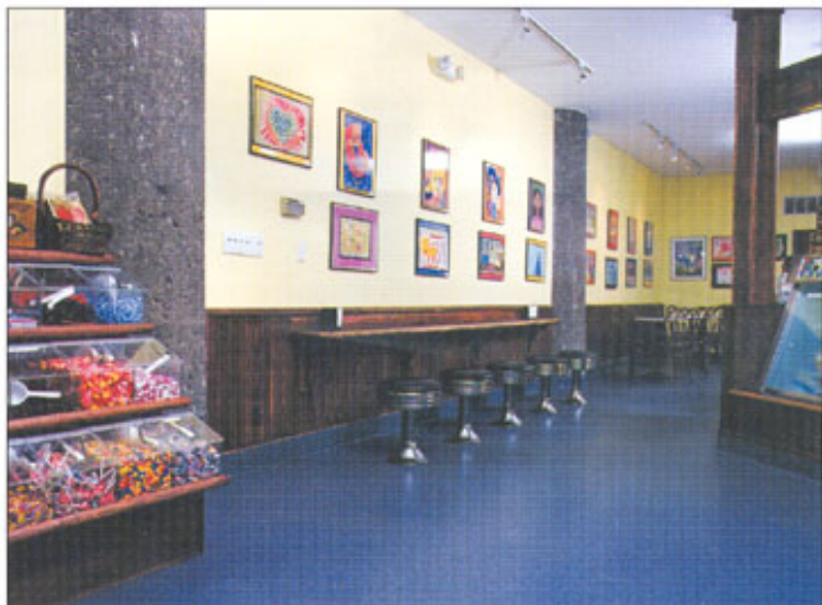
Early epoxy application completed at an ice cream parlor.
